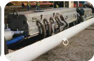
The cleaner and vacuum work in tandem to blast clean, vacuum and recycle grit on each internal field joint.
